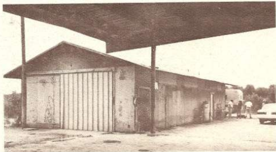
TIPP team inspects a substandard labor camp
